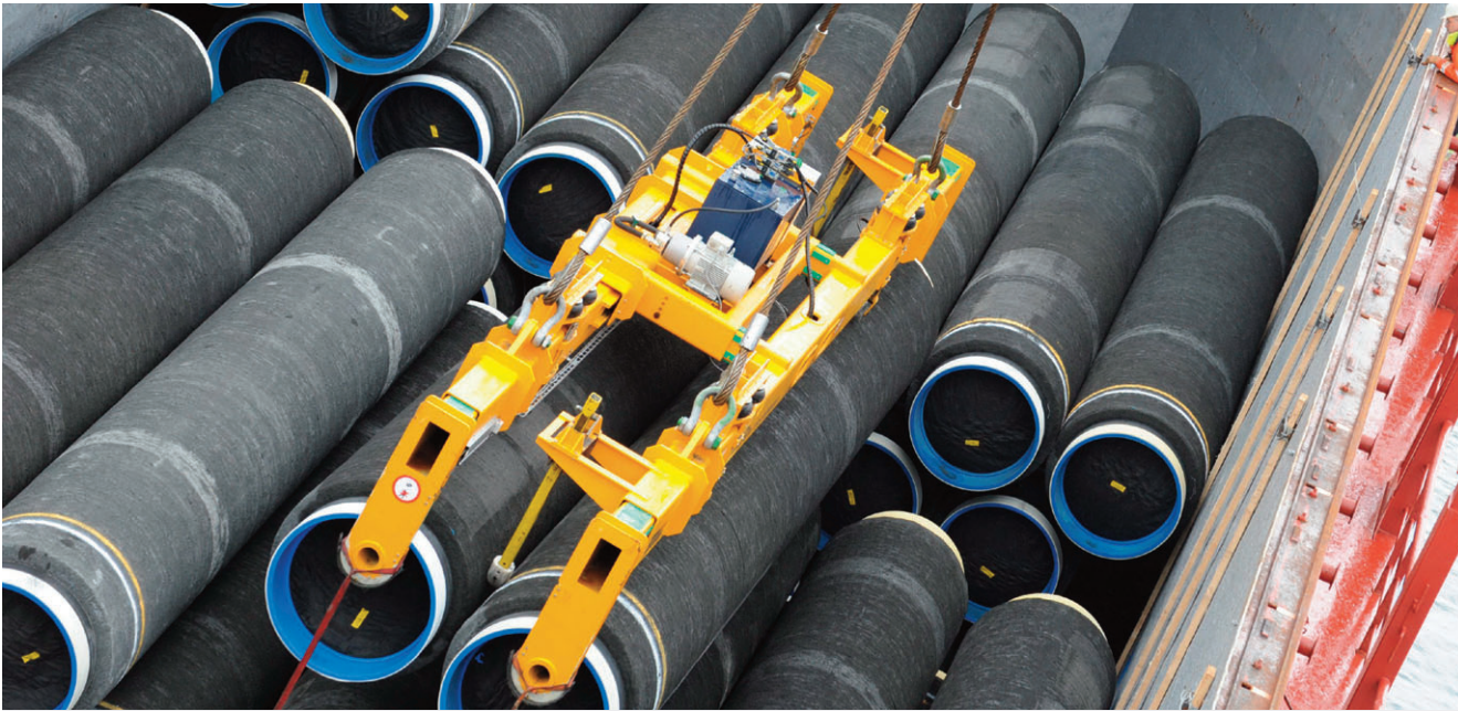
Steel pipelines at Sassnitz-Mukran ferry harbour on the Baltic Sea island of Ruegen being loaded onto a cargo vessel for the construction of the Nord Stream gas pipeline, on 7 October. | ANA/EPA/STEFAN SAUER
